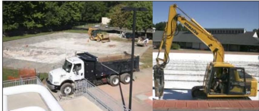
BIG DIG...Demolition of Westfield's Memorial Pool swimming facilities continues on Tuesday. At left, workers have completed the demolition of the kiddie pool. At right, a worker attacks the drained main pool. By yesterday, the interior walls had been pulled into the pool; exterior drain walls were slated to be pulled into the pool yesterday and today.
