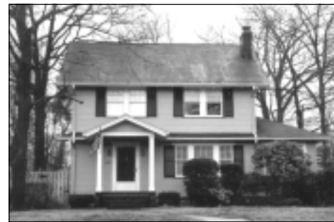
Burgdorff ERA, Realtors, 600 North Avenue West, Westfield is pleased to announce the sale of 651 Raymond Street, Westfield. The property was marketed by Warren Rorden and sold by Elaine Demyen.
