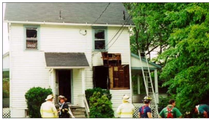
FIRE SCENE...Westfield firefighters survey the damage to a wood frame house at the corner of Palsted Avenue and West Broad Street last Thursday after battling a blaze which broke out in a front office area of the structure. The building is used as office space by the Westfield Community Center, which is headquartered across the street. A preliminary report has ruled the fire accidental.
