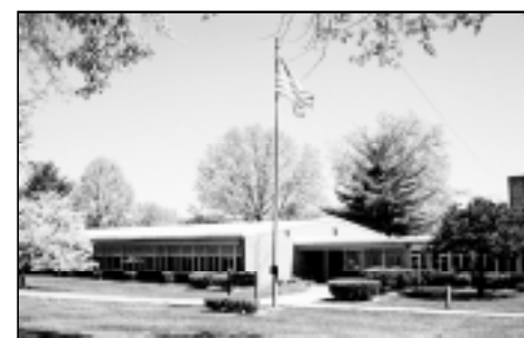
WASHINGTON SCHOOL Circa 1954, additions 1956 and 1993 900 St. Mark's Avenue Connie Odell, Principal (908) 789-4600 http://www.intac.com/~washingtn
