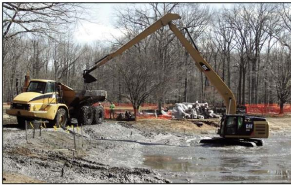
RESTORING THE LAKEBED... Crews at Nomahegan Lake in Cranford continue to remove accumulated sediment from the northern half of the lake. Photo courtesy of County of Union
