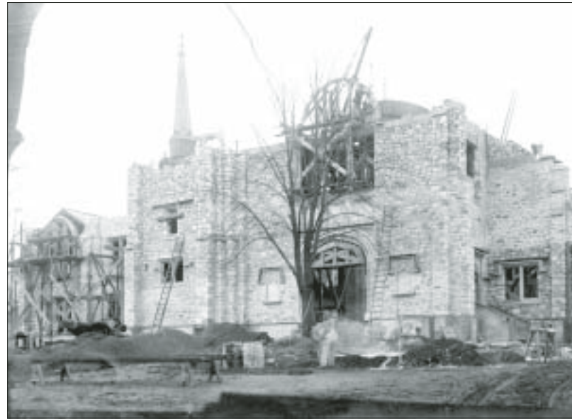
MAKING THE GRADE... This photo of the First United Methodist Church in Westfield under construction is believed to have been taken in 1911. Also standing to the left at the time was the second church, in which the Town Clock originally resided. The clock and bell were removed and hoisted into the new tower using either horse or mule power, pictured at left. The second church, standing on what is now the parking lot, was demolished once the new building was completed. At the time, East Broad Street was at grade level. In later years, an underpass was built to carry the Central Railroad of New Jersey tracks overhead. So, East Broad Street was lowered by several feet to allow passage under the bridge. Thus, the church was elevated to an even higher point, where it rests today on the circle.
