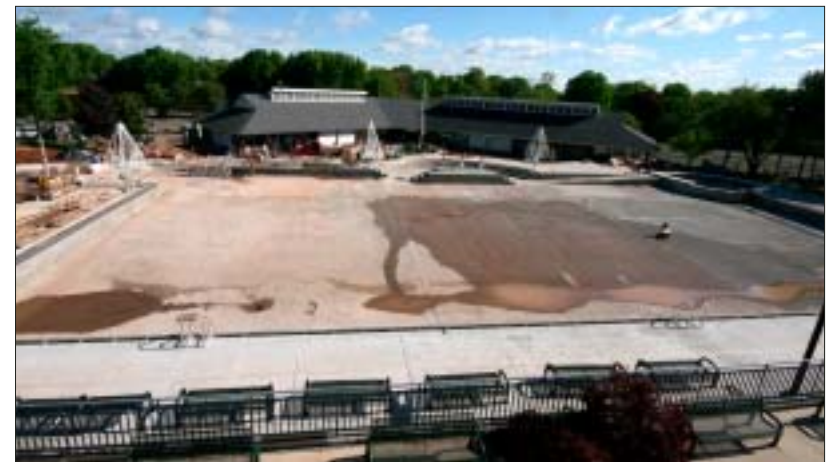
DIVE IN... With just over two weeks to go, the Westfield Memorial Pool is nearing completion. Palm trees are in, water features in the children's pool are ready, and the umbrella stands are in place. The decks are being completed, as are the ramps to the main deck. The adult pool is being power-washed to ready it for tiles and its final coating in the next week. After that, it's a splashing good time.
