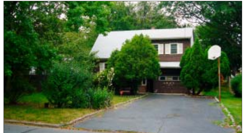
Sara Magnola for The Scotch Plains-Fanwood Times NO ONE'S HOME... This abandoned residence on the corner of Saville Row and Martine Avenue drew complaints from neighbors due to its unsightly appearance and overgrown landscaping, prompting the Borough of Fanwood to send in the Department of Public Works to clean it up. The borough is in the process of acquiring a lien on the property.
