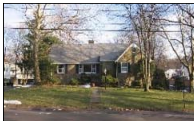
SCOTCH PLAINS $675,000 Open and airy! Wonderful expanded Ranch with open floor plan. Gourmet Kitchen for the cook's delight. A must see home
