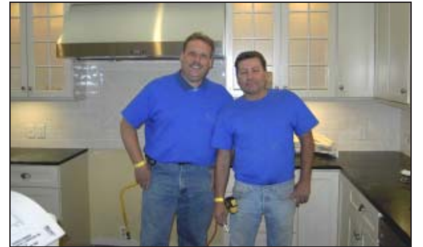
EXTREME MAKEOVER...Friends Brian Zuk, left, and Kitchen Expo's Ron Frank, right, both of Westfield, and Kim Lambertson of Fanwood (not shown) helped install the kitchen that went into the new home of Beverly Turner and her 18 special needs adopted children.
