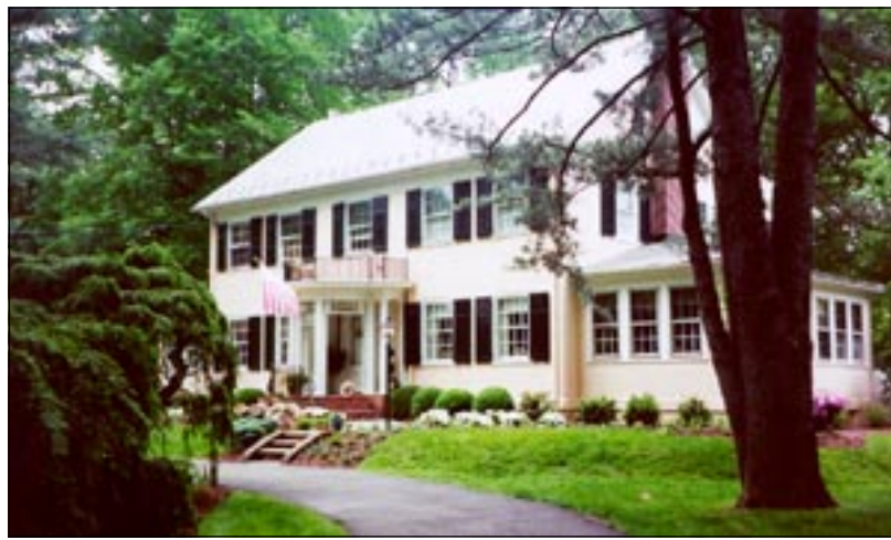
DISTINGUISHED HOMES... The owners of the Westfield home pictured above will be honored tonight, Thursday, June 22, at the Westfield Historic Preservation Commission's Eighth Annual Commendation Awards Reception at 8 p.m. in the Council Chambers of the Westfield Municipal Building. Award recipients will include Mr. and Mrs. Jonathan Baum, the owners of the Georgian Colonial at 720 Lawrence Avenue pictured above.
